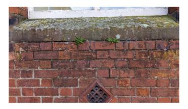
Sandstone blocks and edge stones need repaired or replaced. In a few cases this is cosmetic, but mostly these stones form the first line of defence against the weather, and once compromised, weather damage then increases exponentially.
